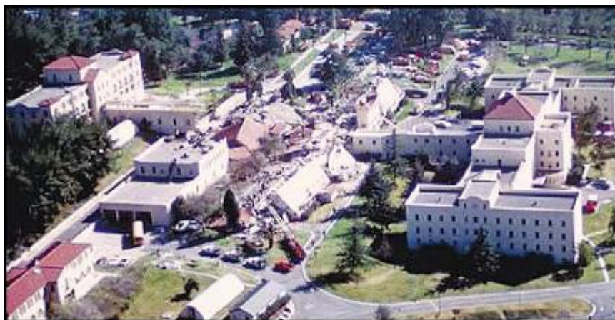
San Fernando Medical Center collapse, 1971
